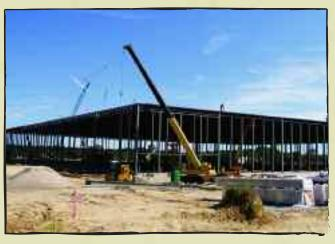
of Fort Wayne, Indiana. The vertical support columns and roof-support structure were fabricated by Helgeson Steel from beams provided by Steel Dynamics. The roof utilizes joists and is covered with steel decking supplied by New Millennium Building Systems. **BELOW** Painted beams prepared by Helgeson Steel, such as those shown in the foreground, form the framework for the large biodiesel facility being erected at Claypool.
